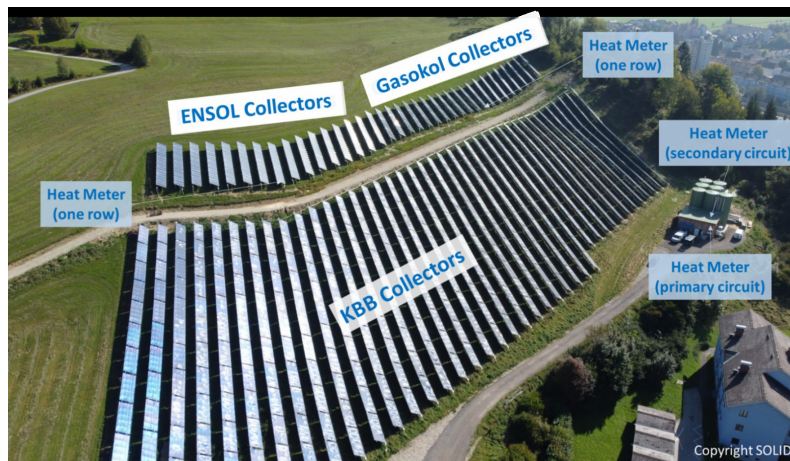
Figure 59. Picture of Solar District Heating plant in Mürzzuschlag showing the different collector fields and the installed heat meters. Source: SOLID.
